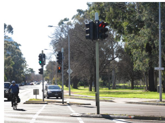
Existing crossing and slip lane on the eastern side of Glen Osmond Road at the intersection with Hutt Road with poor waiting areas and high speed vehicle turning movements
